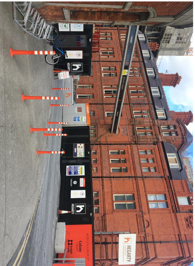
Vehicle Entrance at RGRE Spencer Place South
