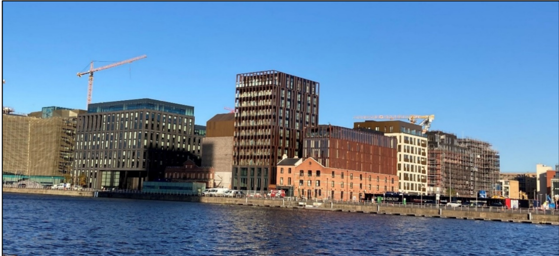
Figure 2.6: View of the Dublin Landings site (Central Bank to the left) from Sir John Rogerson's Quay, showing City Block 9 to the right. (Source: TPA, November 2020.)
