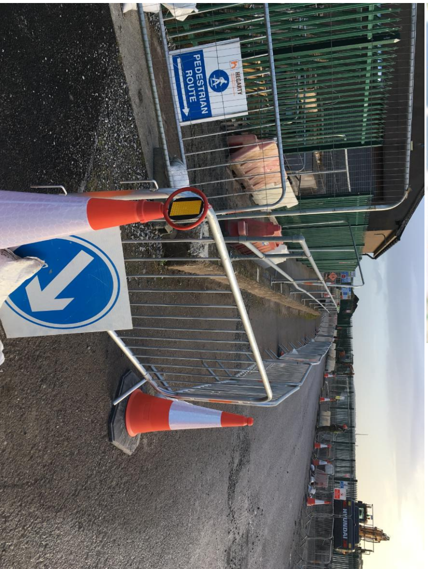
Typical Pedestrian Crossing Point & Pedestrian Route Separated from Vehicles Route
