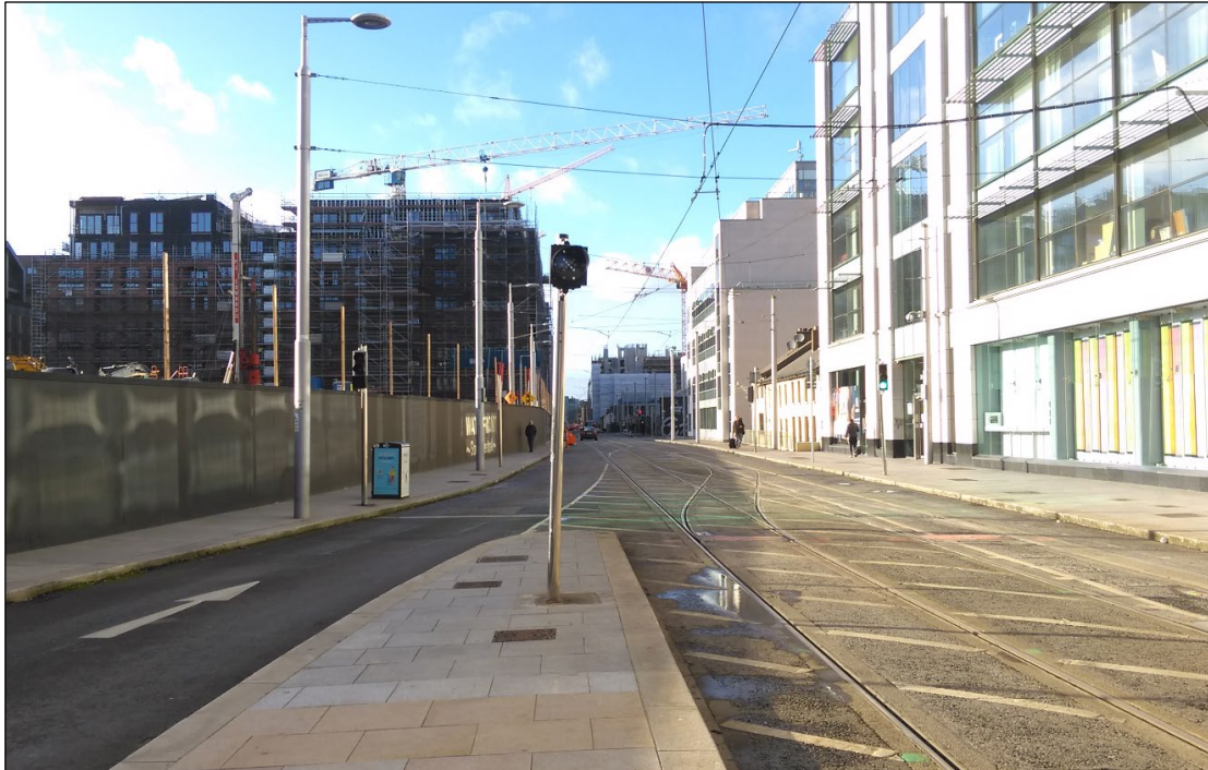
Figure 2.3: View of northern site boundary, looking west along at Mayor Street Upper. (Source: TPA, November 2020.)
