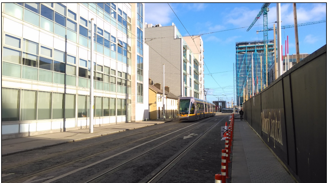
Figure 2.12: Photograph of Luas tram exiting Point Village Luas Station along Mayor Street Upper. (Source: TPA, November 2020.)
